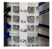
Figure 2 - Typical Control Wire Terminals for a Utility-to-Generator Setup
