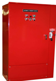
Fire Pump Transfer Switch
